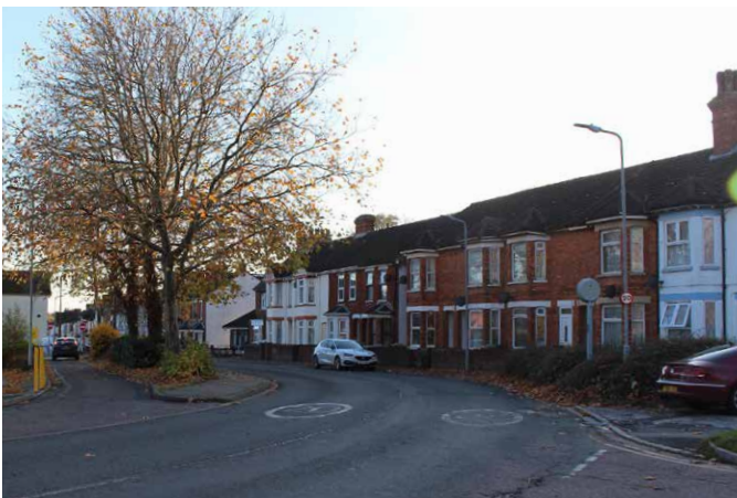
Typical Victorian terrace alongside town centre
